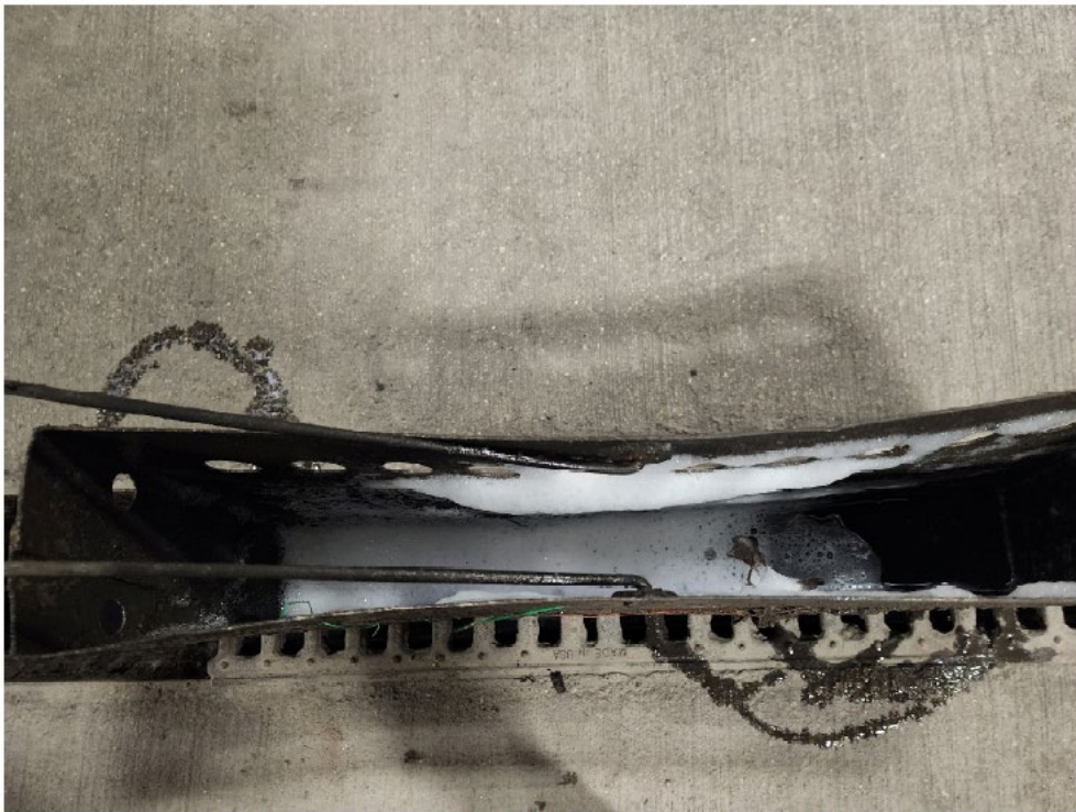
Trench Drain Sediment Bucket After Running Spray Nozzles
