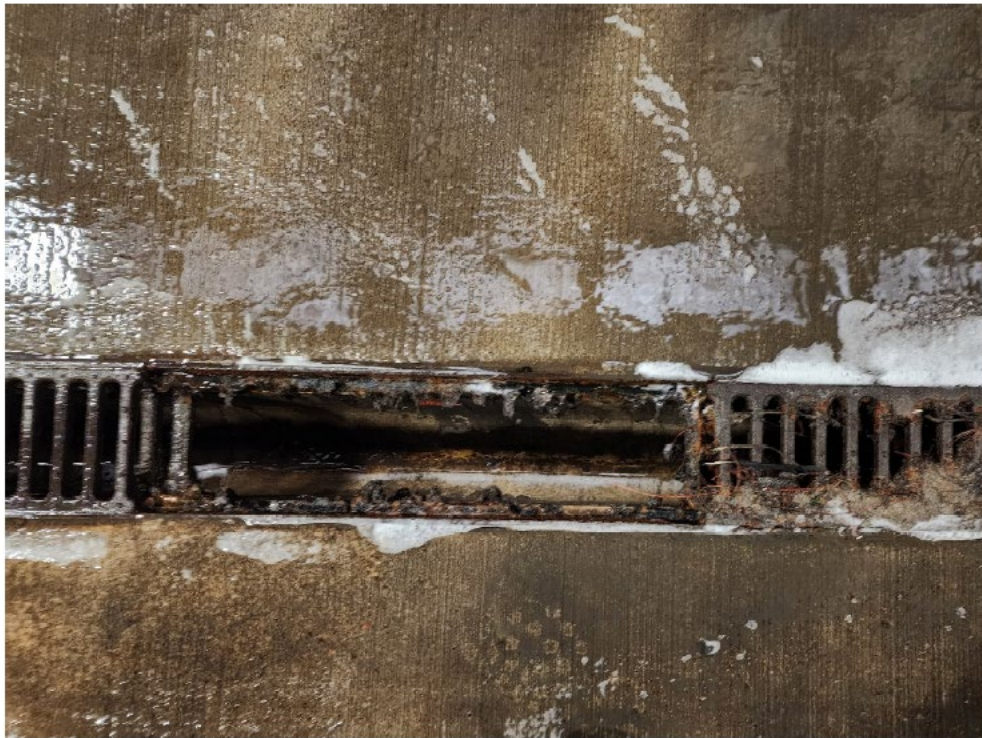
Trench Drain After Running Spray Nozzles
